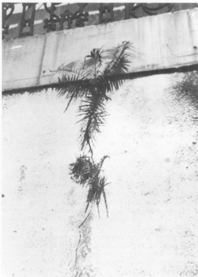
Fig. 12. (a) Water intrusion caused by rusting metal, or (b) plant growth left unattended will gradually enlarge these cracks, resulting in spalling, and eventually requiring extensive repair of the stucco. Photos: National Park Service Files.
