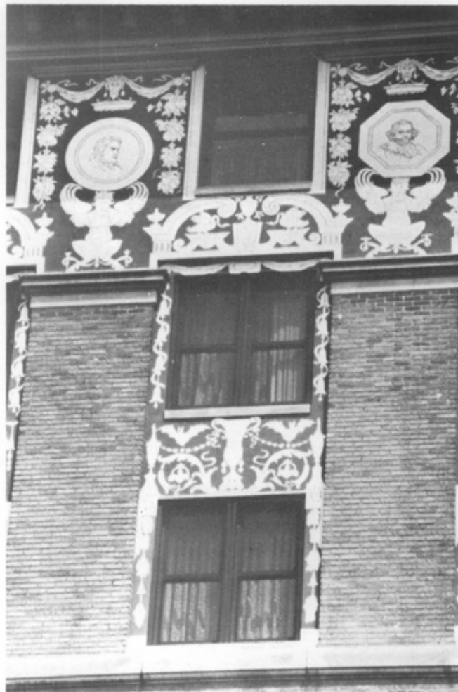
Fig. 11. The Hotel Washington, Washington, D.C. (1916–1917), is notable for its decorative sgraffito surfaces. Stucco panels under the cornice and around the windows feature classical designs created by artists who incised the patterns in the outer layer of red-colored stucco while still soft, thereby exposing a stucco undercoat of a contrasting color. Photo: Kaye Ellen Simonson.
