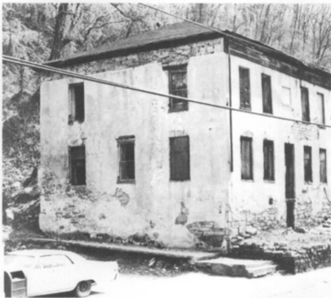
Fig. 7. Patches of stucco have fallen off this derelict 19th century structure exposing the rough-cut local stone substrate. The missing wood entablature on the side and the rough wood lintel now exposed above a second-floor window, offer clues that the building was stuccoed originally. Photo: National Park Service Files.
