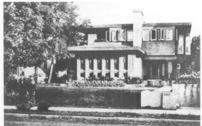
Fig. 3. The William Gray and Edna S. Purcell House, Minneapolis, Minnesota, was designed in 1913 by the architects Purcell and Elmslie in the Prairie style. Stuccoed in a salmon-pink, sand (float) finish, it is unusual in that it featured a 3-color geometric frieze stencilled below the eaves of the 2nd story. The Minneapolis Institute of Art has removed the cream-colored paint added at a later date, and restored the original color and texture of the stucco. Photo: Courtesy MacDonald and Mack Partnership.
