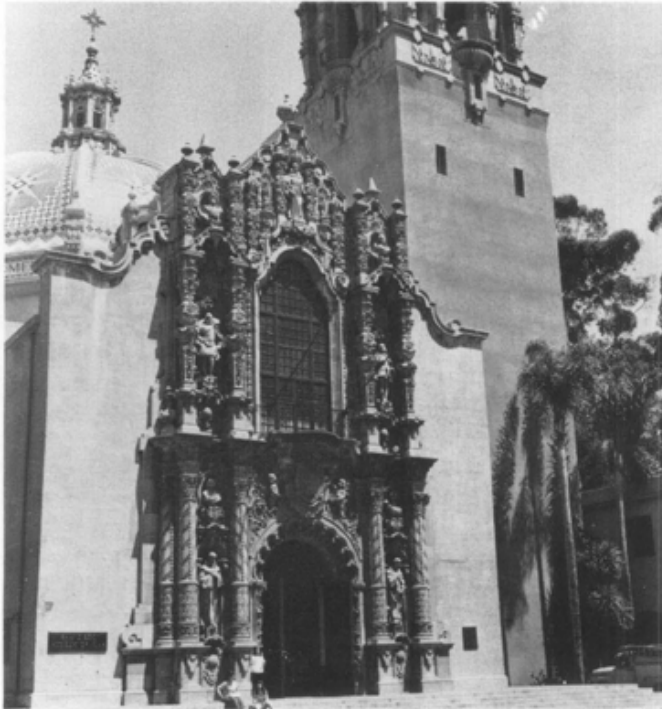
Fig. 4. The elaborate Spanish Colonial Revival style of this building designed by Bertram Goodhue for the 1915 Panama California Exposition held in San Diego's Balboa Park emphasizes the sculptural possibilities of stucco. Photo: C. W. Snell, National Historic Landmark Files.
