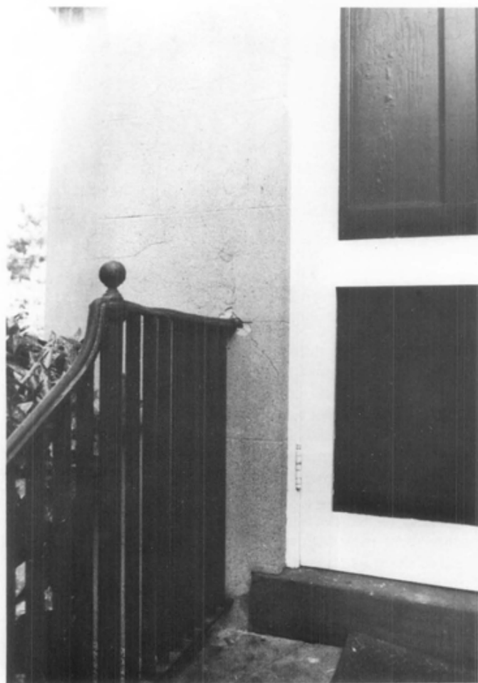
Fig. 12. (a) Water intrusion caused by rusting metal, or (b) plant growth left unattended will gradually enlarge these cracks, resulting in spalling, and eventually requiring extensive repair of the stucco. Photos: National Park Service Files.
