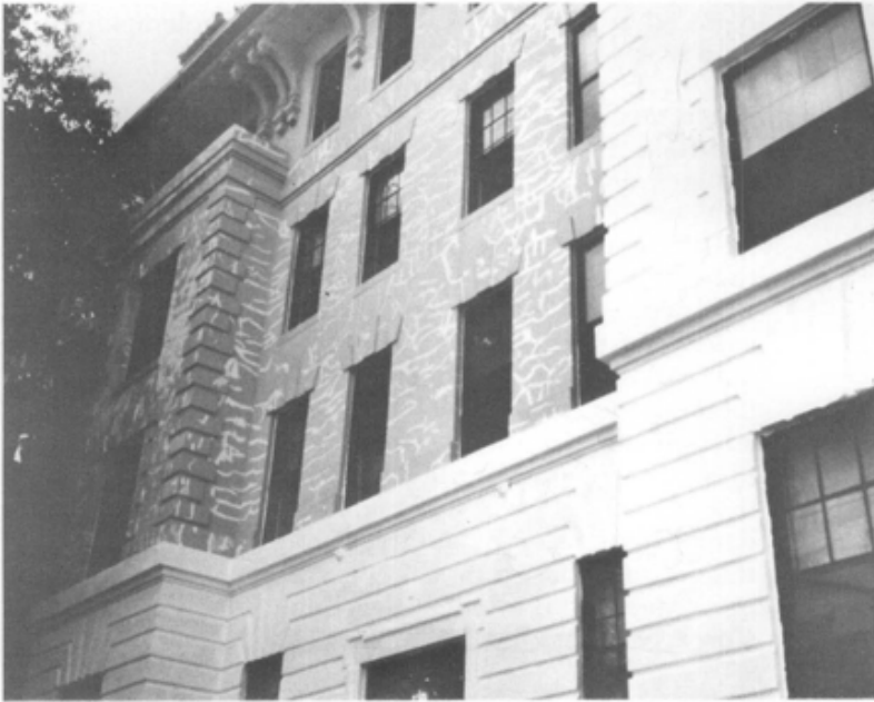
Fig. 13. (a) In preparation for repainting, hairline cracks on this Mediterranean style stucco apartment building were filled with a commercial caulking compound; (b) dirt is attracted and adheres to the texture of the caulked areas, and a year after painting, these inappropriate repairs are highly obvious. Photos: Anne Grimmer.
