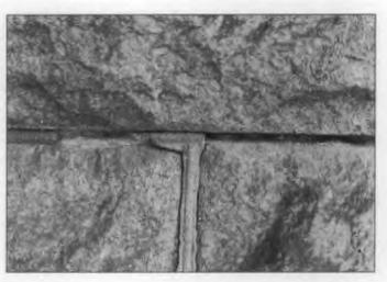
Figure 8. Due to inadequate joint preparation, the repointing mortar has not adhered properly and is falling out of the joint. Photo: Robert C. Mack, FAIA.
