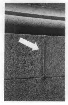
Figure 7. The dark stain on either side of the vertical joint on this sandstone watertable probably resulted from the use of a bonding agent that was not properly cleaned off the masonry after repointing. Photo: Anne Grimmer.
