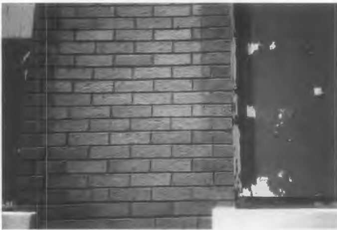
Figure 18. The glazed bricks in the center of the pier were covered by a signboard that protected them from being damaged by the sandblasting which removed the glaze from the surrounding bricks.
