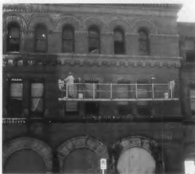
Figure 12. A mild acidic cleaning agent is being used to clean this heavily soiled brick and granite building. Additional applications of the cleaner and hand-scrubbing, and even poulticing, may be necessary to remove the dark stains on the granite arches below. Photo: Sharon C. Park, FAIA.
