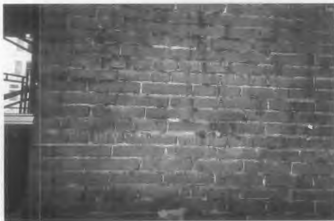
Figure 13. Sometimes it may be preferable to paint over a thick asphaltic coating rather than try to remove it, because it can be difficult to remove completely. However, in this case, many layers of asphaltic coating were removed through multiple applications of a heavy duty chemical cleaner. Each application of the cleaner was left to dwell following the manufacturer's recommendations, and then rinsed thoroughly. (As much as possible of the asphalt was first removed with wooden scrapers.) Although not all the asphalt was removed, this was determined to be an acceptable level of cleanliness for the project.
