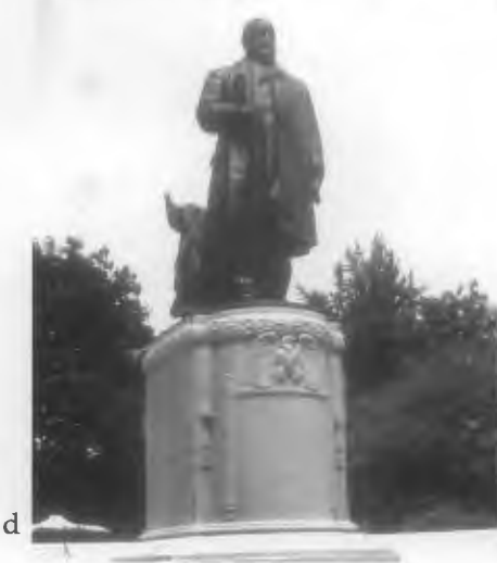
Figure 16. (a) The limestone base was heavily stained by runoff from the bronze statue above. (b) A poultice consisting of copper stain remover and ammonia mixed with fuller's earth was applied to the stone base and covered with plastic sheeting to keep it from drying out too quickly. (c) As the poultice dried, it pulled the stain out of the stone. (d) The poultice residue was removed carefully from the stone surface with wooden scrapers and the stone was rinsed with water. Photos: John Dugger.
