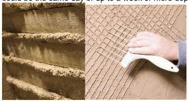
This coat takes up any shrinkage and may crack. You need only worry if the plaster becomes detached from the background. Overworking this coat with the steel trowel can cause it to become detached.
