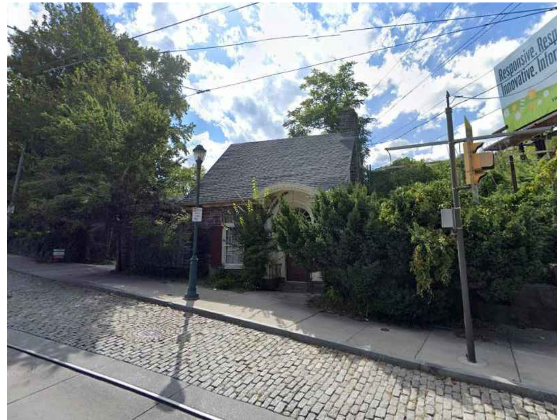
② EXISTING ENTRY CARRIAGE HOUSE 2
